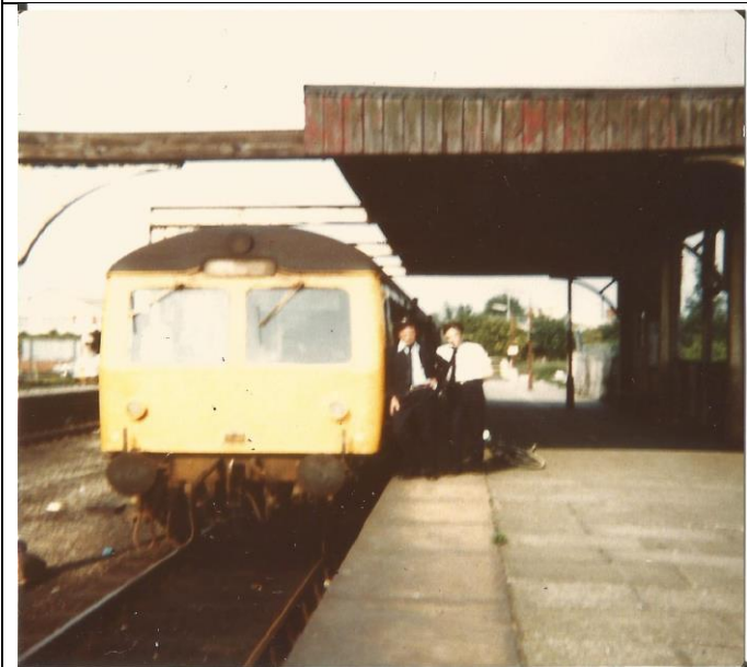
1981 The old St John's remnant station at Bedford. The route to the East ERTA believes should go this way. Rebuilding the old station would be questionable if it prohibited linking round to Bedford Midland from the East as well as the West!
